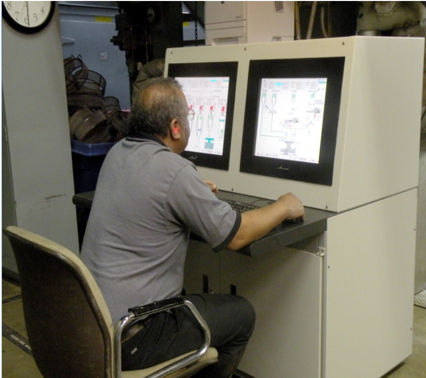
Blank Front Panels on turret provided for panel mounted screens added by customer
