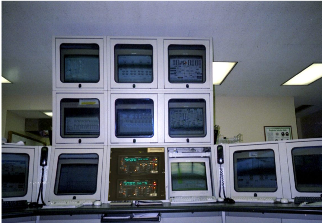
Tier 1on center turret above is equipped with 19in. EIA Racks for process control equipment.
