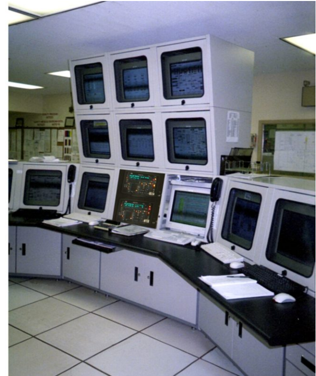
Note that turn angle front panels can be used to mount phones or radios.
