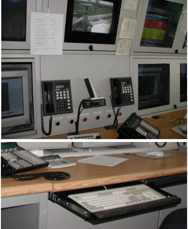
Computer desk shown with Keyboard Tray and blank front panels for phones & operator console controls.
