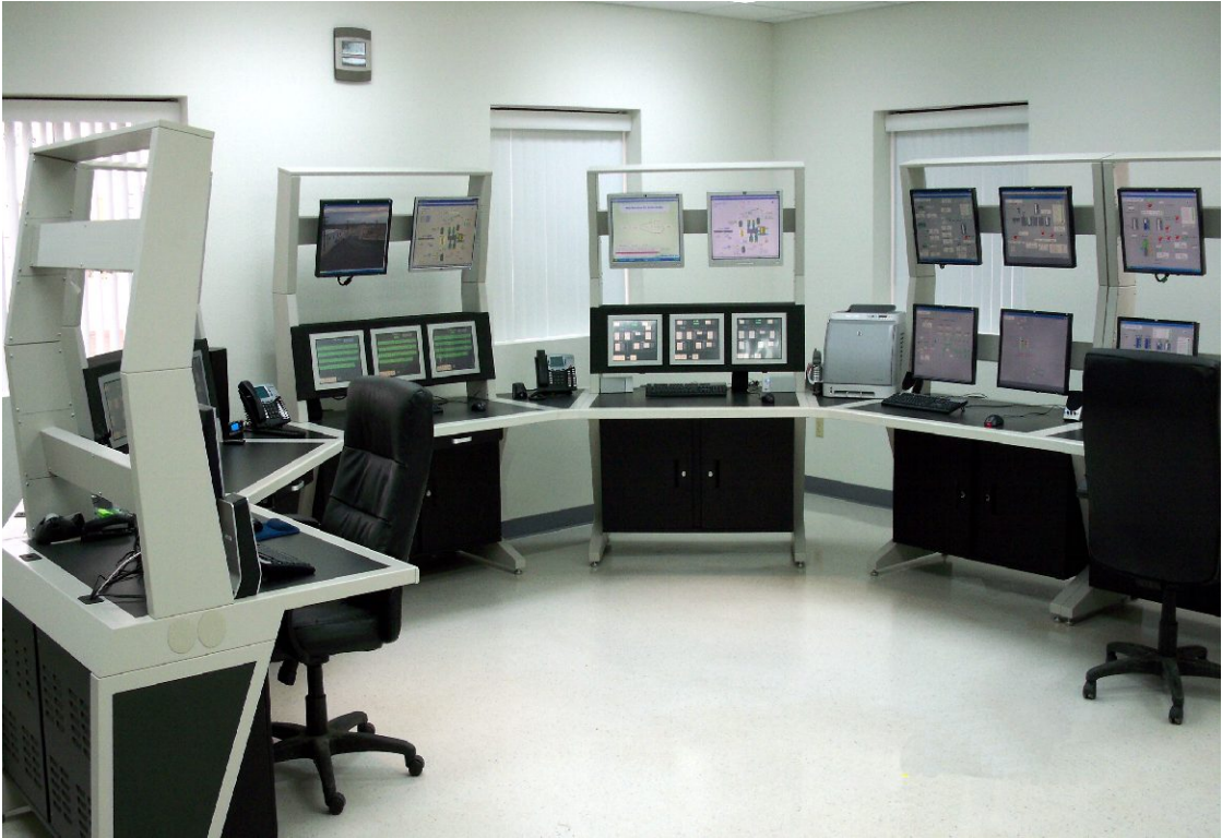
Control Room Design Assistance was provided at no charge. Several options were explored with detailed AutoCAD drawings provided in order to meet operations requirements in U-shaped layout.
