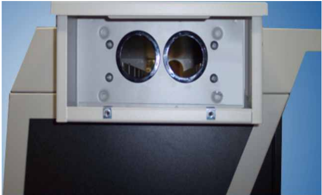
Factory mounted conduit entry box shown closed in top photo Hoffman box opened in lower shot shows horizontal wire way access
