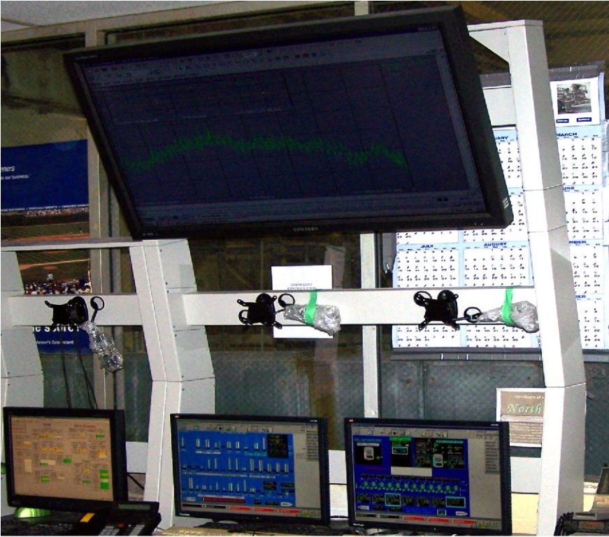
46in. LCD screen was elevated above tier - 2 with 5in. Biscuit Riser option
