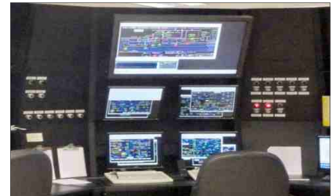
3-Tier 45 Degree Wedge Turrets, Shallow Depth for HMI Workstations on each side of 48 in. monitor tiers
