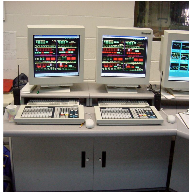
3.5in. high Monitor Riser Shelf; DCS keyboards in front, QWERTY keyboards in back
